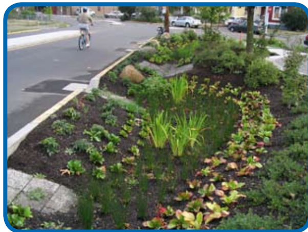
A rain garden is a shallow, landscaped depression that collects and manages stormwater.
