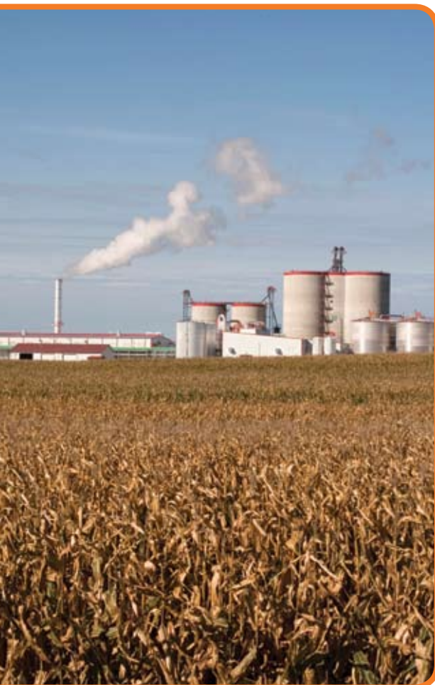
An Iowa ethanol plant
