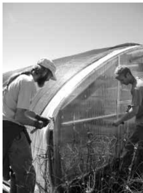
Northwoods employees installing insulation.
