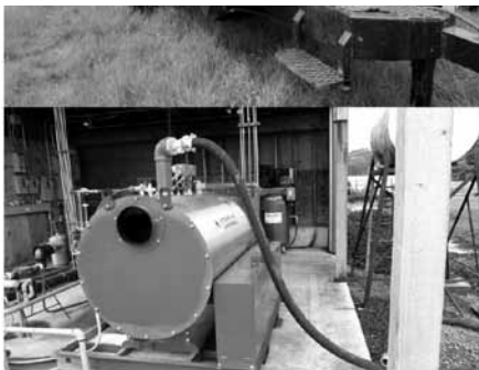
Soil cleaning steam system: trailer and steam generator system
